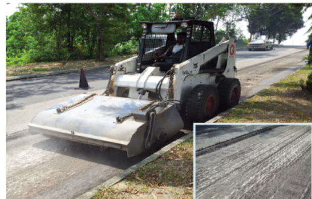
FIGURE 3. Milled pavement is cleaned by mechanical power broom to remove the dust left behind on the pavement. Small figure at the bottom right corner shows the texture of the milling
